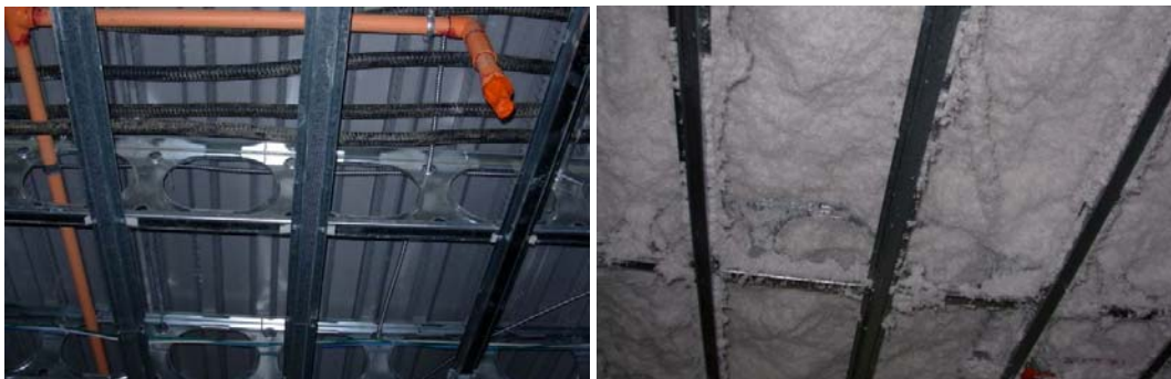
Overhead Thermal and Acoustic Treatment
