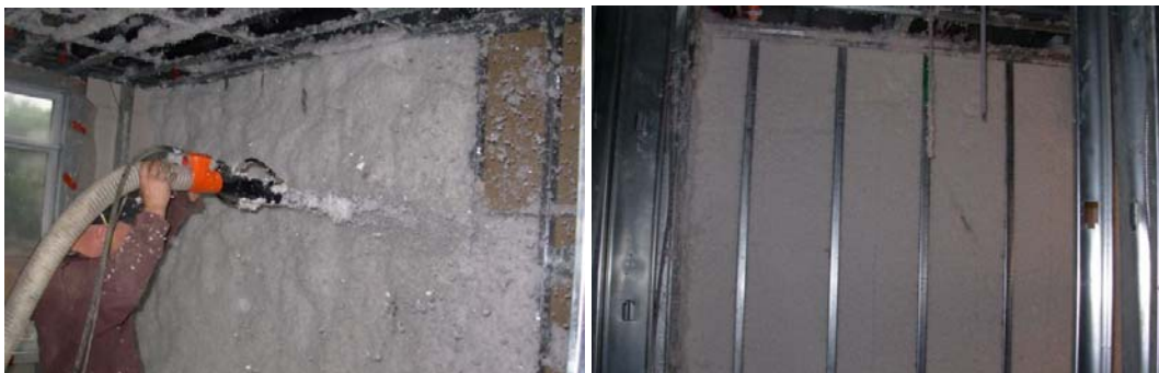
Steel Stud Wall with Gypsum Sheathing
